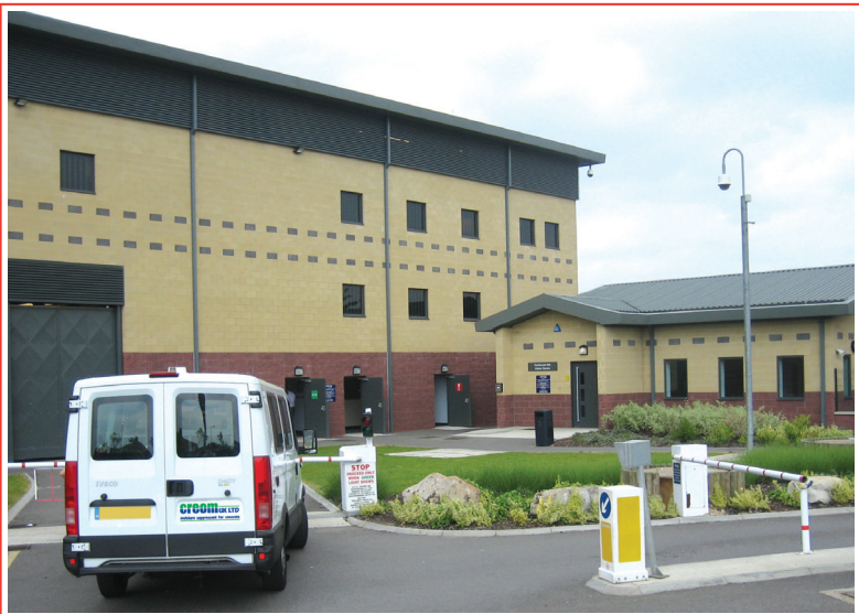
■ Immigration Return Centre - Heathrow 10,000 m2 Fast Track completion using Creom throughout. Finished Floor coverings: Forbo Nairn Marmoleum and Safestep, Flotex and Heckmondwyke Carpet tiles.
